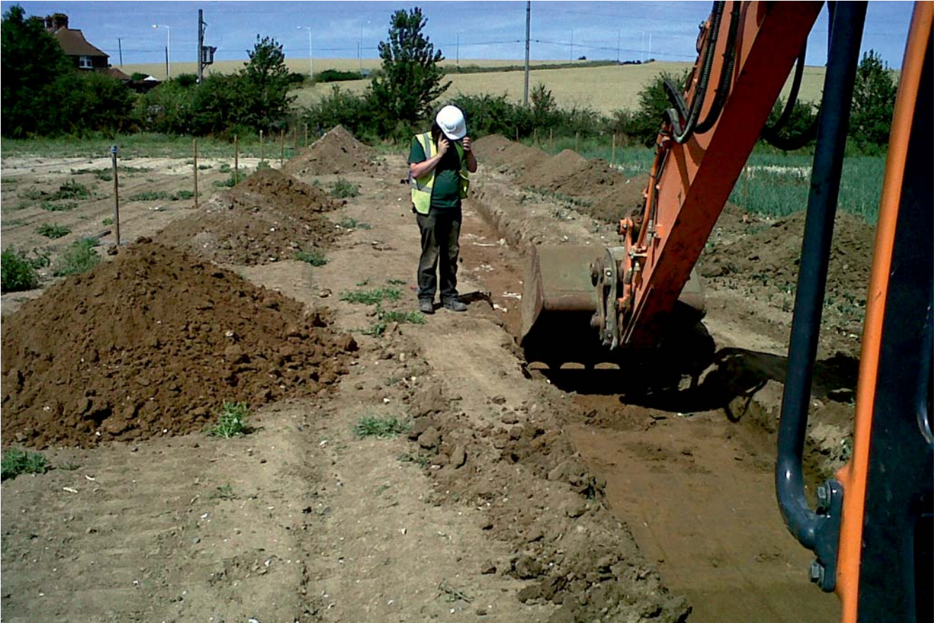
Plate 13. Excavating the pipeline trench just north of Monkton Road Farm.
