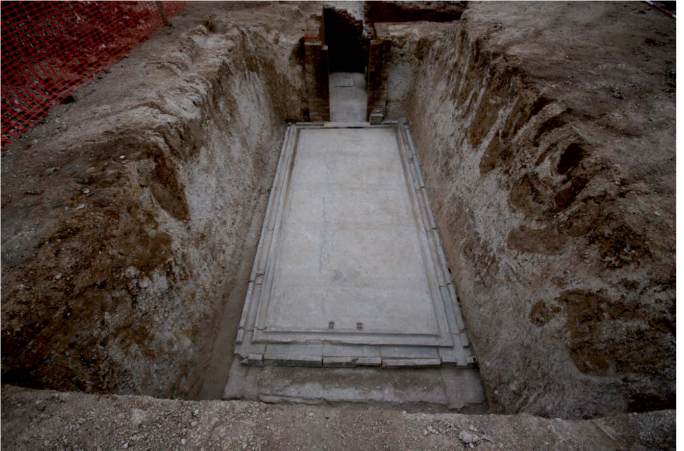
Plate 345. Second World War Structure 61 (G4096). Detail of Room 2, looking east, showing scars on concrete floor.
