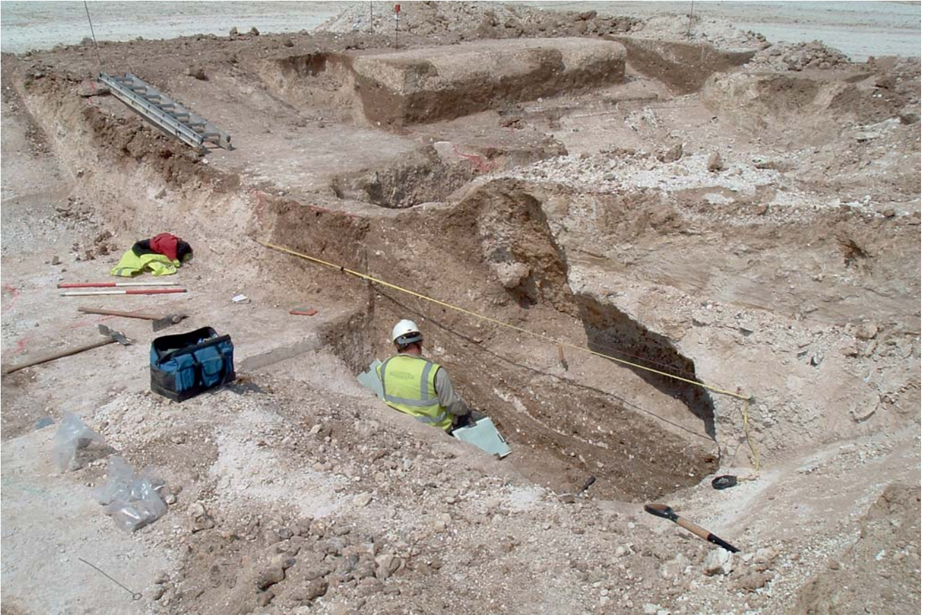
Plate 241. Excavation of underground chambers (G2040 & G2161), showing one of the underground chambers half-sectioned, looking north-east.
