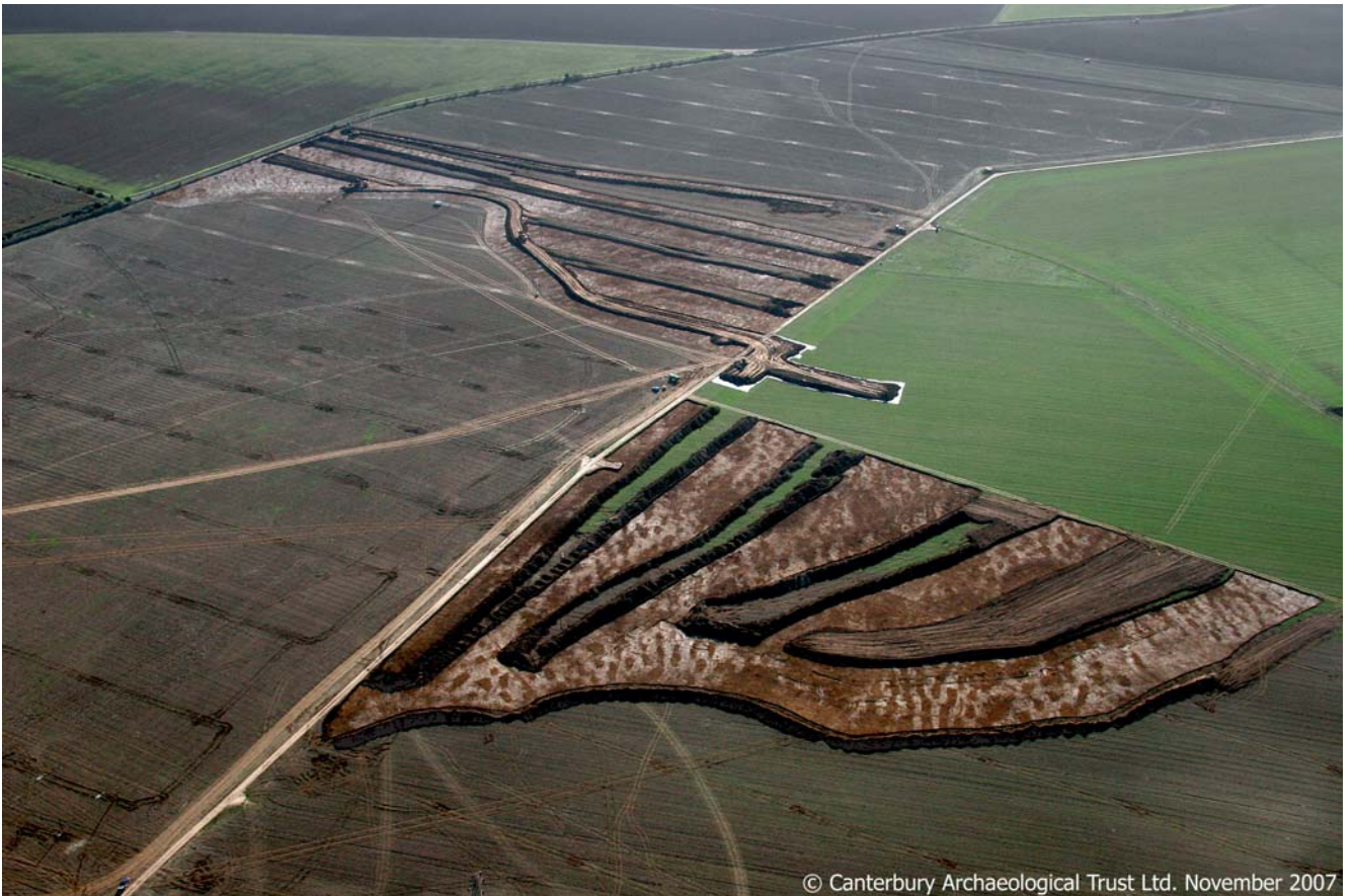
Plate 4. Topsoil strip of Plateaus 2 & 4 looking south-east.
