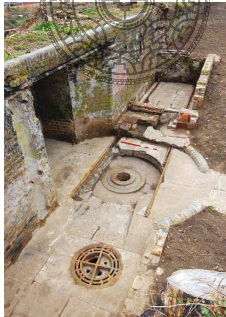
▽ Fig 4.20. Vertical Lift Emplacement following investigation, looking north-east (scale 1m).
