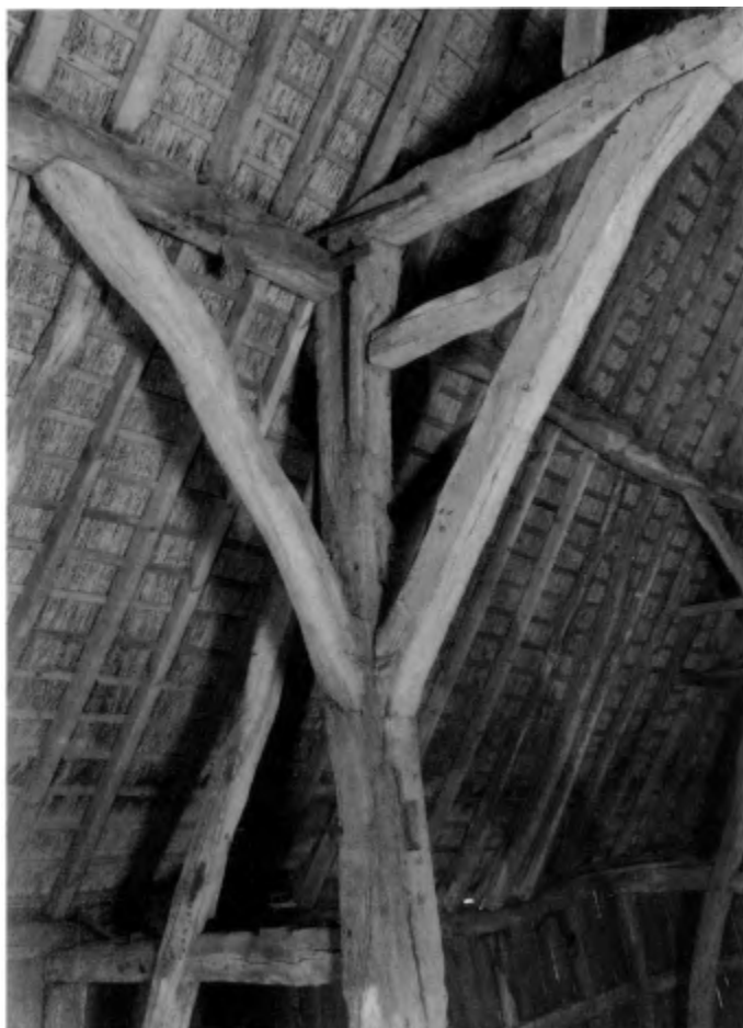
Main post assembly. South-east elevation showing spandrel strut.
