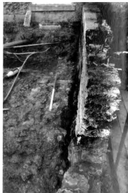
Crack between medieval arch and post-medieval parapet wall. Scale: 1 m.
