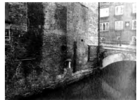
The riverside wall of King's Bridge House showing mill fabric including a brick roundel possibly indicating the position of the westernmost mill wheel.
