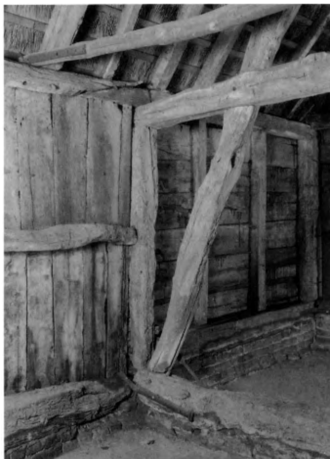
Detail of south-east aisle-wall showing reverse assembly.
